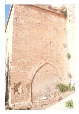
Diagonal fissure above arch indicates subsidence and/or seismic effect
